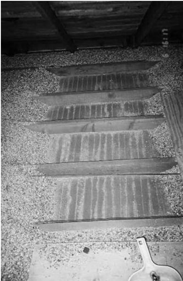
Figure 8—View of Zonolite in attic after moving by homeowner method.
