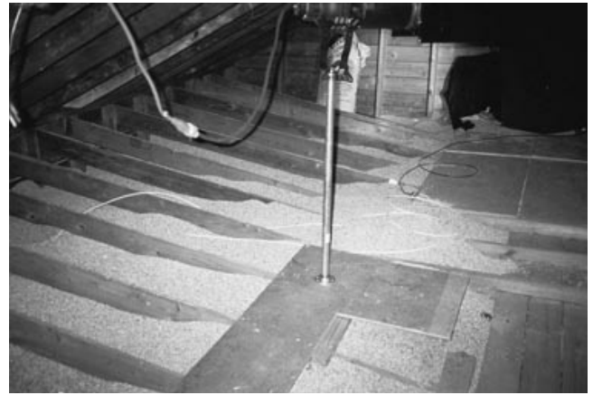
Figure 5—View of attic in home C.
