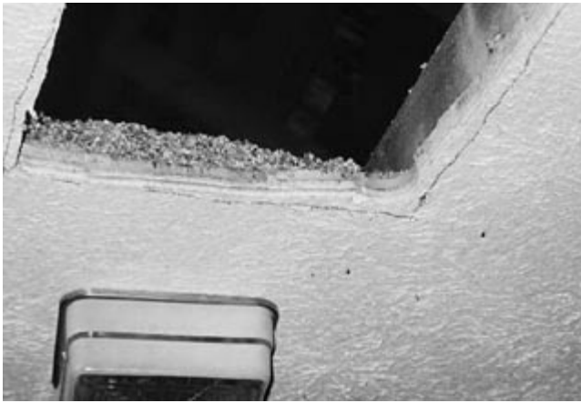
Figure 6—View of ceiling after cutting, home A.
