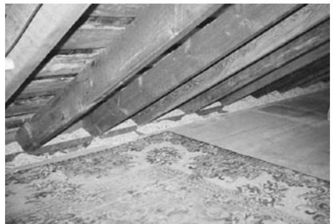
Figure 9—View of ZAI at top of wall cavity before shop vacuum removal.
